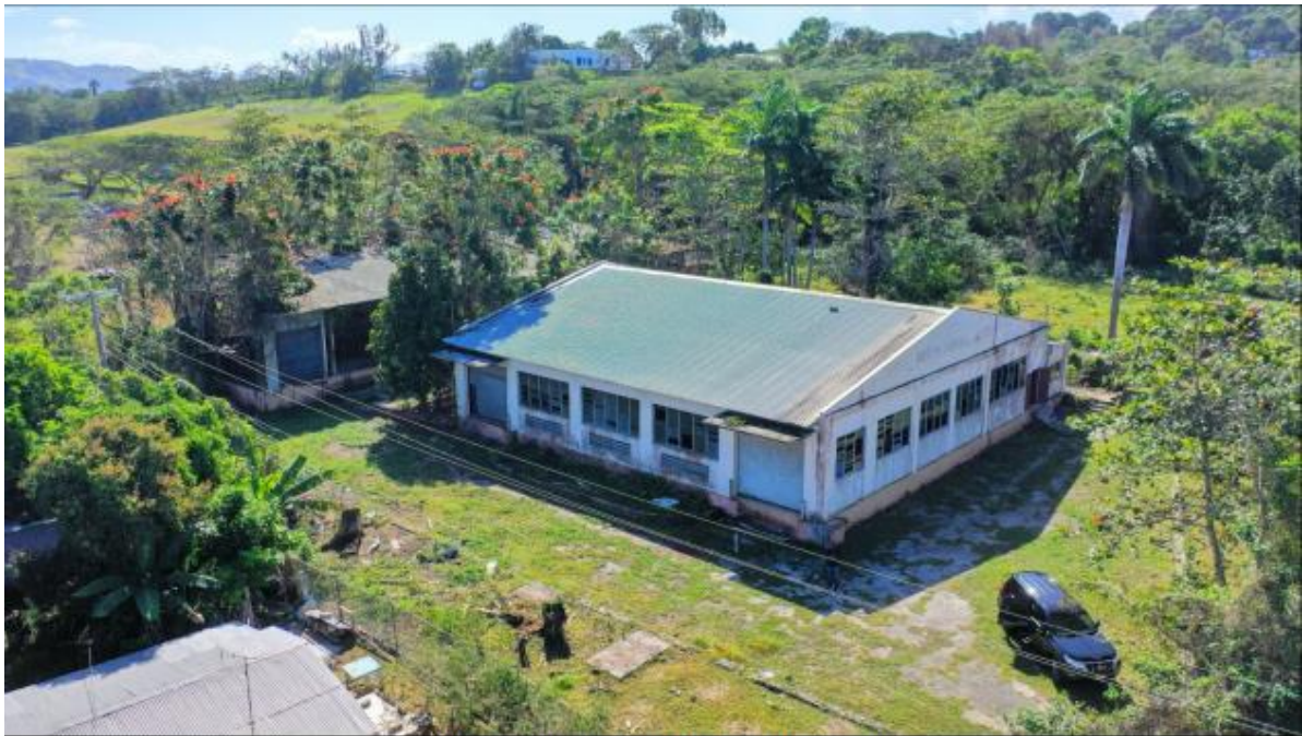
View of the building facing south east
