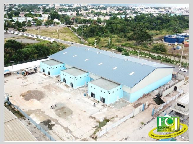
Phase 1 of the **Garmex Free Zone Redevelopment and Expansion Project** is almost completed. Four buildings totalling 90,000 sq.ft. are now operational, with the exception of the sewer works which are currently being connected along with some minor defects to the buildings. With the connection of the sewer being done, the buildings are being prepared to be handed over to their new clients shortly.
