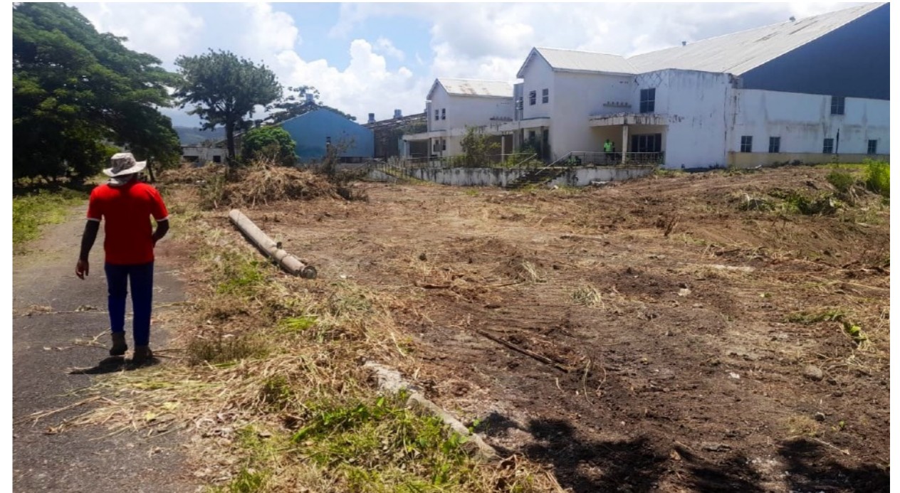
Excavation of the existing structure to be done
