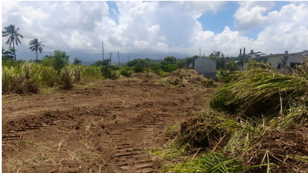
Excavation of the land being done
