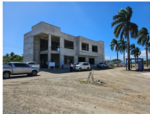
The NCB building located on Block A – 75% complete.
