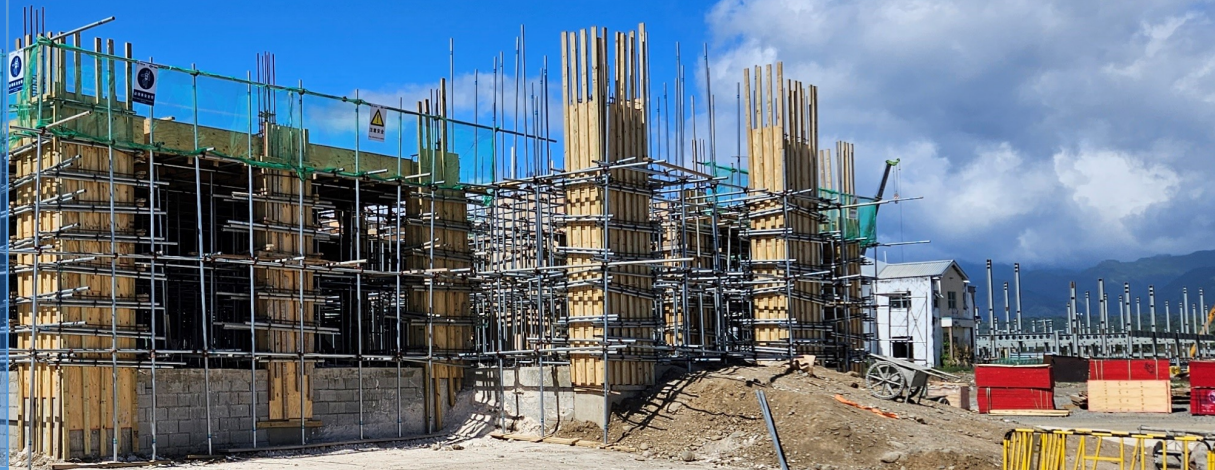
The St Thomas Municipal Corporation building located on Block B – 55% complete.
